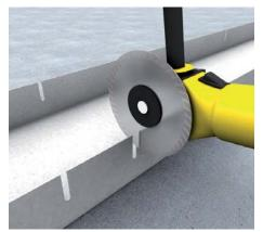
**13 | Slotting** If needed, add slots to the duct bottom piece, then burr and galvanise the joints.
