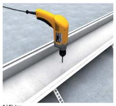
**5** | **Fixing** Mount duct to the rough concrete in two places per length using plugs.
